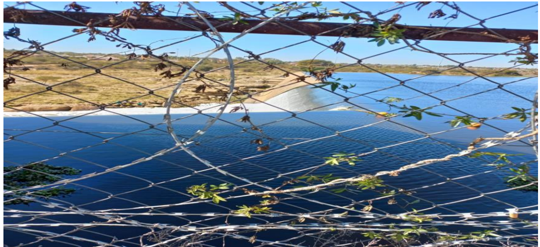
Figure 4: The photo depicts an estuary of Leeuwkraal Dam, which is an abstraction reservoir for Temba WTW at the time of inspection.
